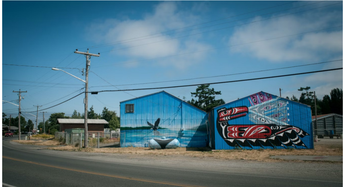
Murals painted onto storage buildings located in Lummi Nation Port Authority (Emtman, 2014).
