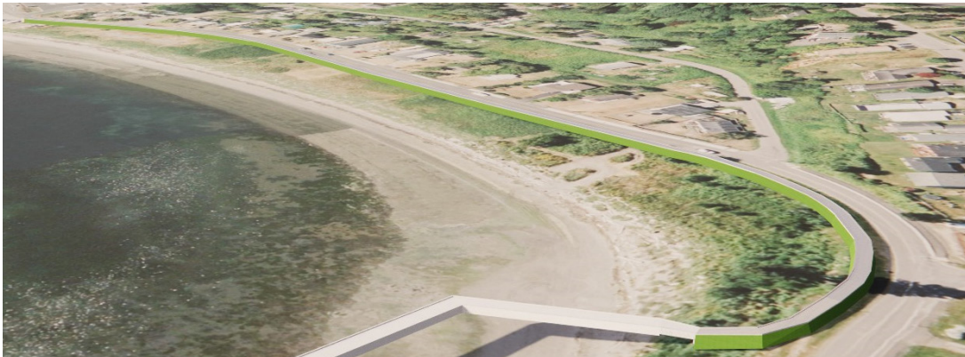
Figure 4.5. Aerial view of berm structure.
