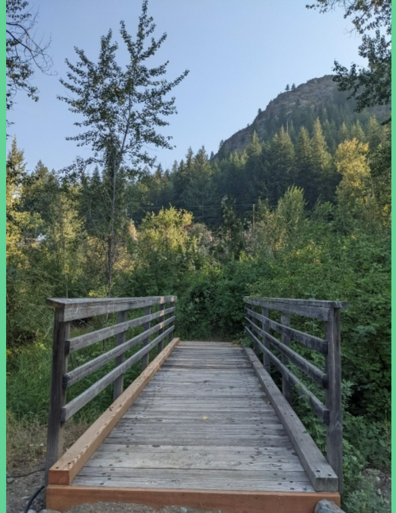
Bridge at Twisp Ponds site
