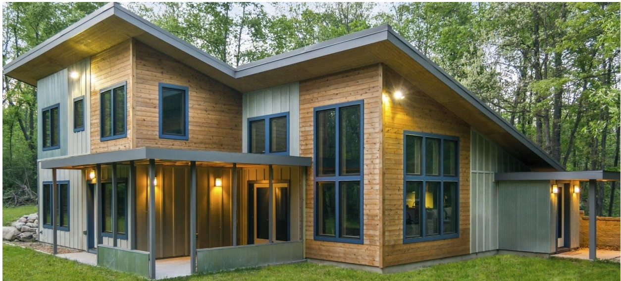
South-facing passive-solar home.
