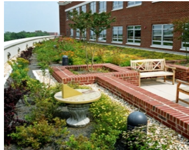
INTENSIVE GREEN ROOF
