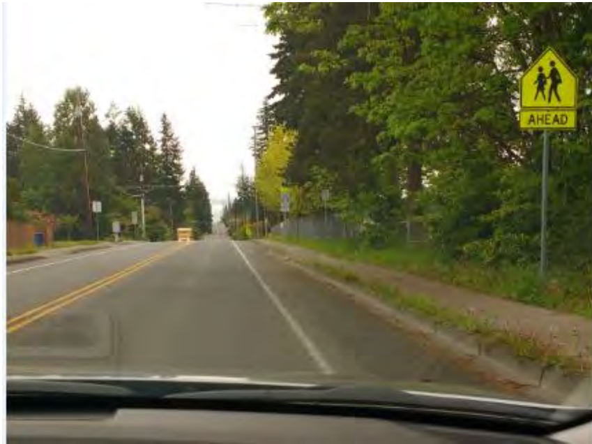
Image 1: This image looks east on 220th St on the north side of Westgate Elementary. The picture shows a crosswalk sign, a clear bike lane, and the start of the school zone. The picture also shows the sidewalk on the South side of the road, which is perceived to be “too narrow.” Not shown is the electronic speed limit sign to the west, or the hill that one has to drive up to get to this spot.
