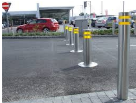
An example of retractable traffic bollards for our pedestrian and bike boulevard alternative.
