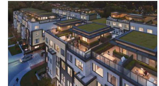
Figure 8.31 “The Vic Towns” in North York, on Victoria Park Avenue in Toronto, ON. (Source: the Solotex Corporation).
