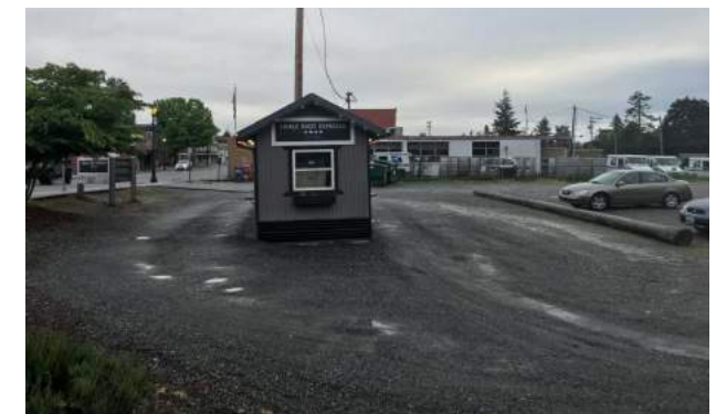
Figure 8.22: 540 North Olympic Avenue - parcel #00529900900101 (May 2020)
