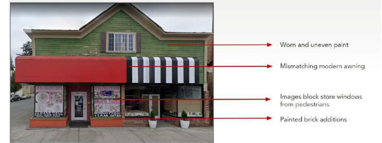
Figure 4.13: An example of a building in downtown that does not meet the historic design standards, this building has since been improved.
