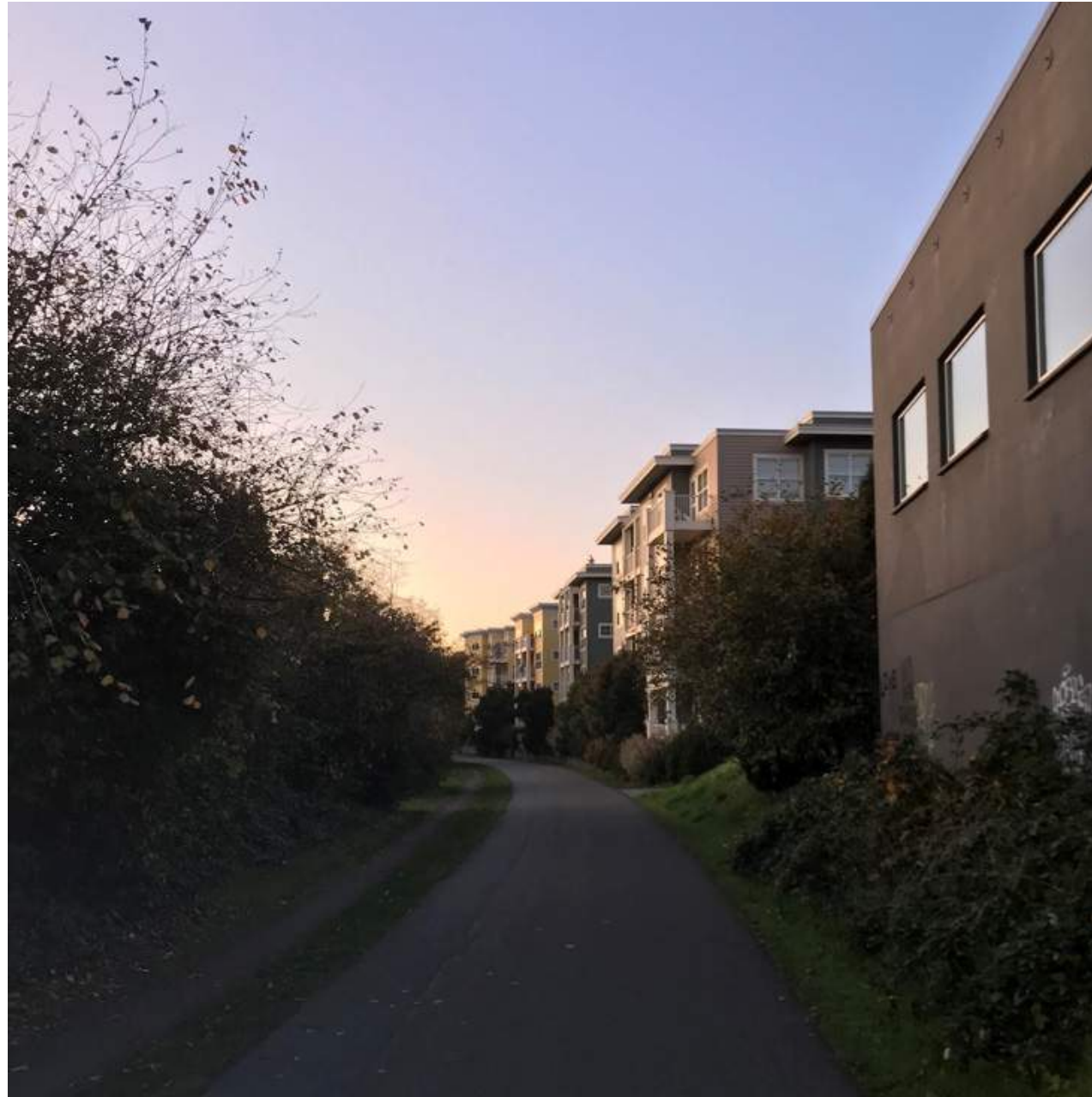
Figure 5.35: Residential Development on the Interurban Trail (Seattle, WA.)
