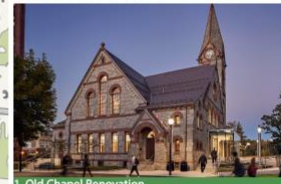
1. Old Chapel Renovation
