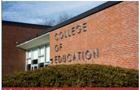
5. Furcolo School of Education Renovations
