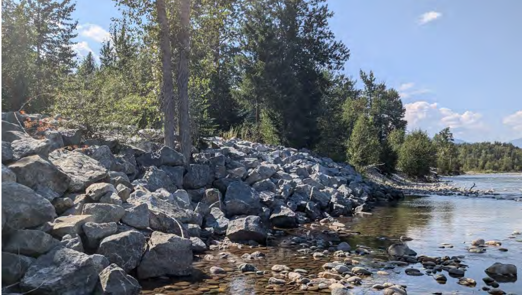
Photo from Ava Donelan of the Riprap on the Methow River on Whittaker's land
