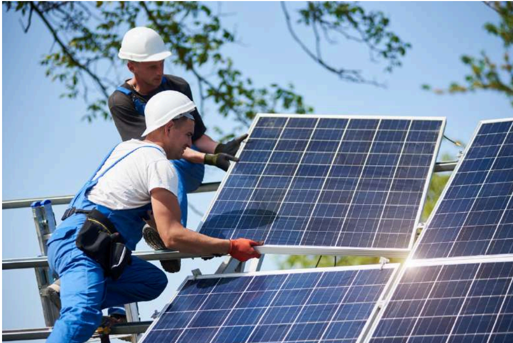
Construction on solar panel [Photograph] anotoliy_gleb. Adobe Stock
