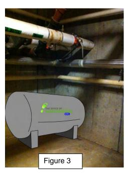
the pump back up to the main pipes and restrooms, then back down. Pipes would also need to be connected from the catchment tank and pump up to the rest of the plumbing pipes towards the ceiling (Morrow 2013). See figure 3.
