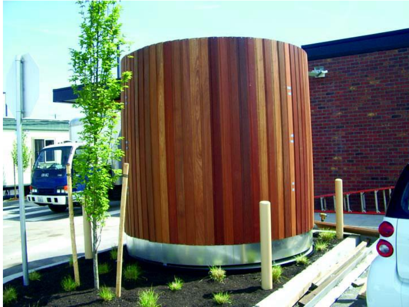
Figure 3 shows a galvanized metal tank that is covered with a visually pleasing, stained wood siding.
