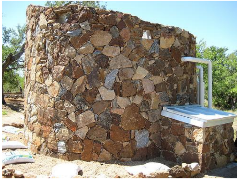
Figure 5 shows a rock wall built around a 10,000 gallon tank in order to blend in to the natural settings. The proposed tanks could incorporate something like this using brick to match Western overall architectural theme.
