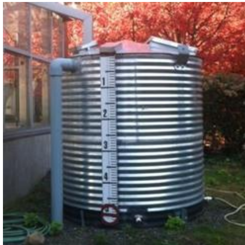
Figure 2 shows an educational metering system located on a 1,000 gallon tank next to the Biology greenhouse.
